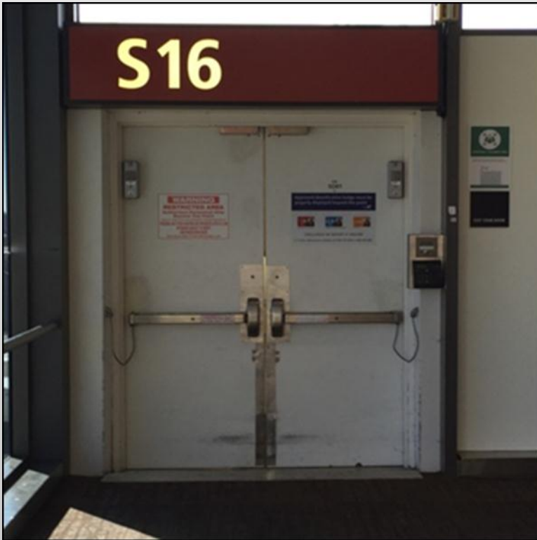
Current door portals
